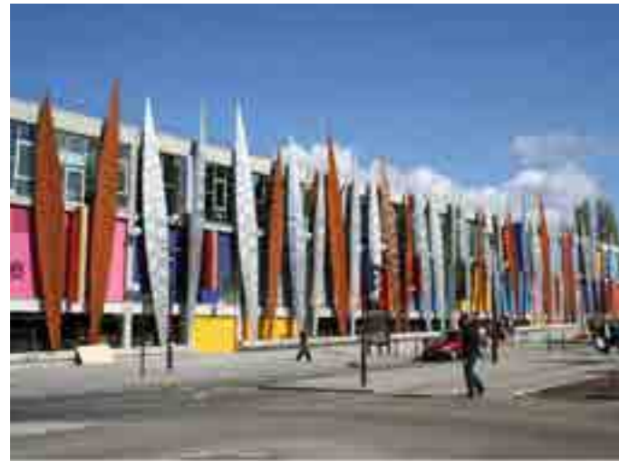
Parking silo simple, Beaulieu, Nantes
